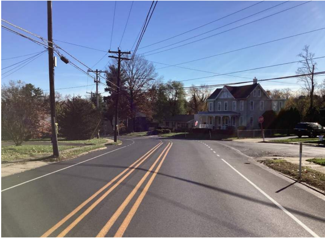
Direction / Road: Wb. Route 513 Approach / Departure: Approach Distance: 50 feet
