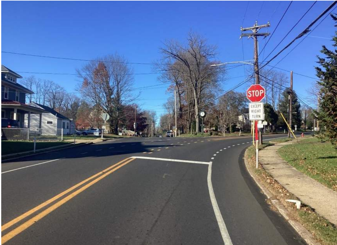
Direction / Road: Nb. Route 513 Approach / Departure: Approach Distance: 50 feet
